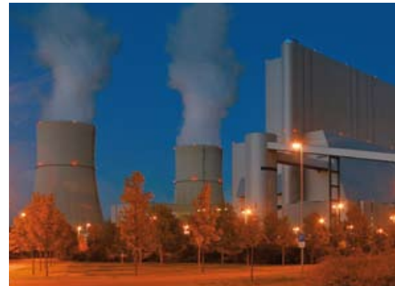
Natural-draft cooling tower of the 'Schwarze Pumpe' coal-fired power plant in Germany with an output of 2 x 800 MW.
